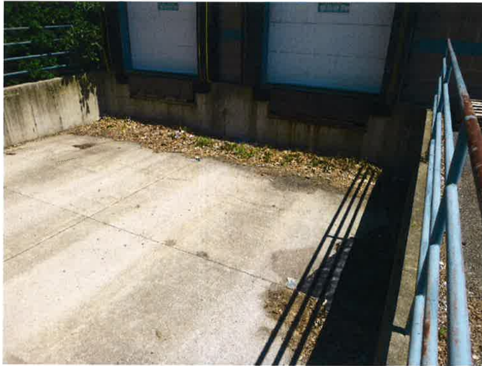
13: View of the french drain observed in the sunken loading dock on the western side of the building on the subject property, facing east.
