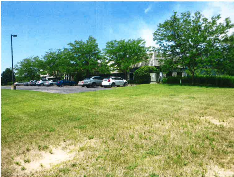
12: Exterior southeast corner of the building on the subject property, facing northwest.
