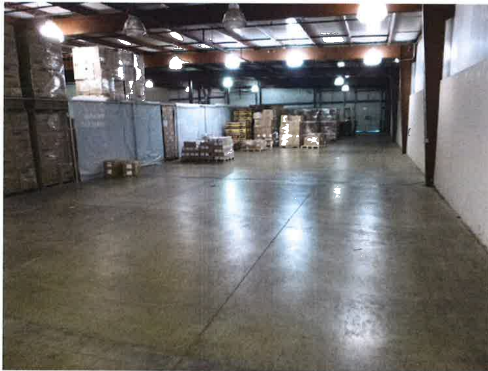
18: Interior view of the warehouse portion of the St. Clair Apparel portion of the building on the subject property, facing west.
